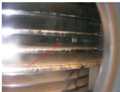
Picture D / damaged kieselguhr cake after emptying
