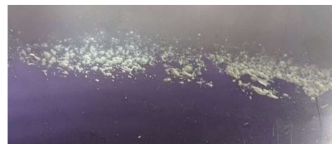
Chlorobutyl ring of inner wall of tank
