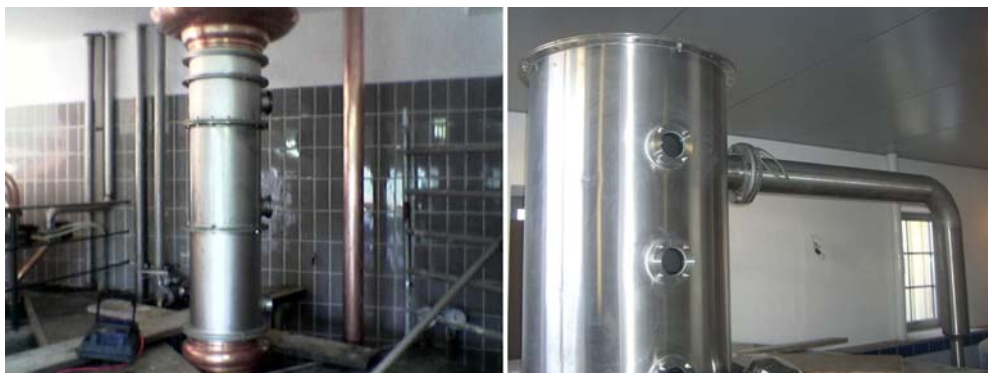
Figure 3. Examples of retrofitted rectification wort-boiling systems (left: nostalgic; and right: modern).
